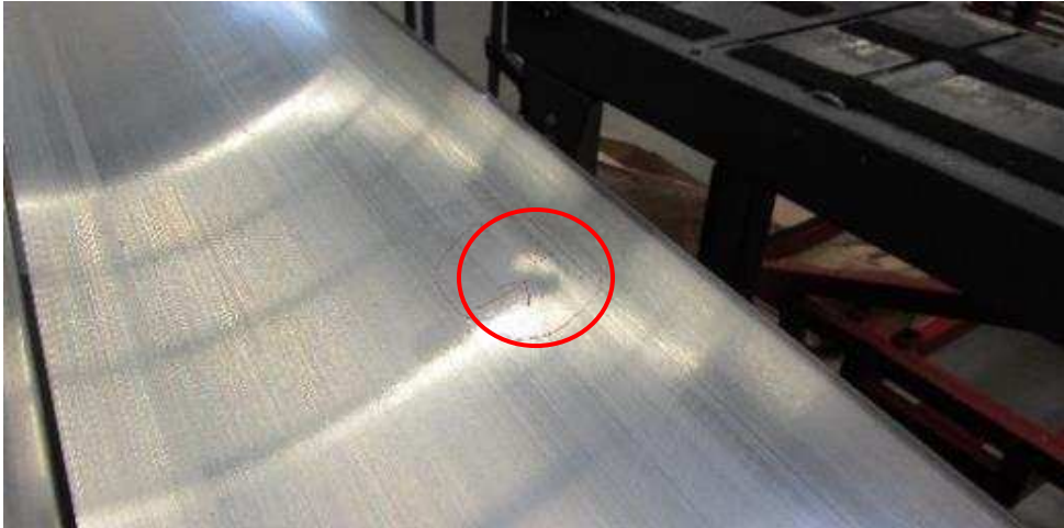
Figure 5 – dent in surface
