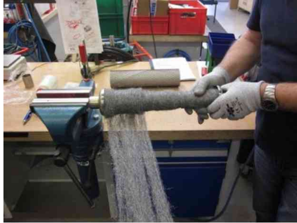
Fig. 4 - Installation of wool
