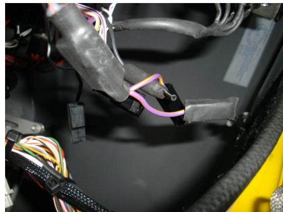
Fig. 4 - Isolation of cable end
