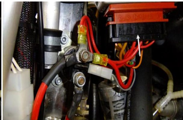
Fig. 2 – Cable connector on rectifier-regulator
