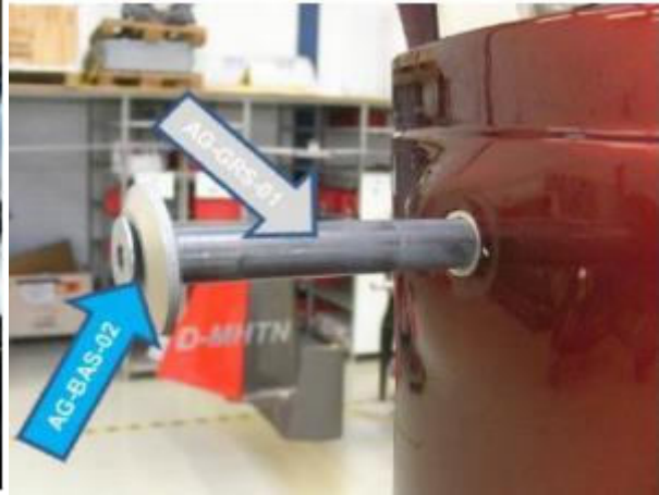
Fig. 3 - Installation of mast pins
