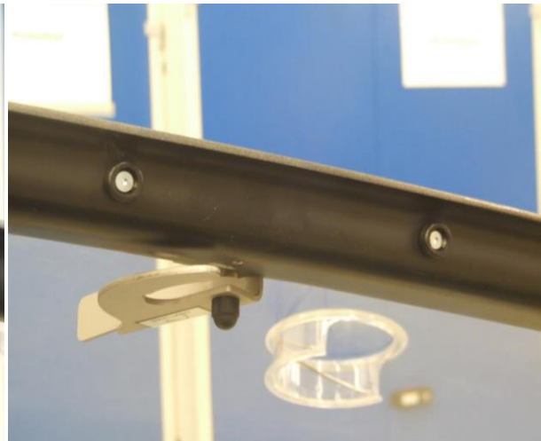
Fig. 4 - Canopy spacers installed
