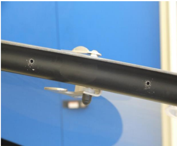
Fig. 3 - Attachment bores drilled
