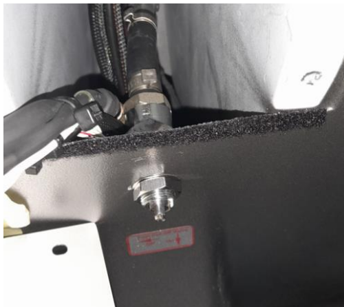
Figure 26: New shut-off valve installed
