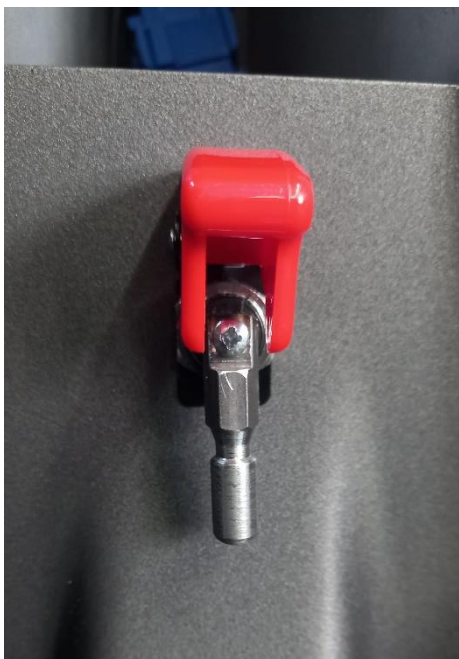
Figure 28: new shut-off installed in open position
