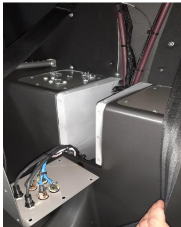
Figure 2: Intercom Panel removed
