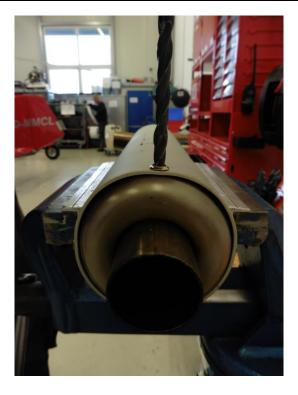
Fig.3: Drill out the rivet pin
